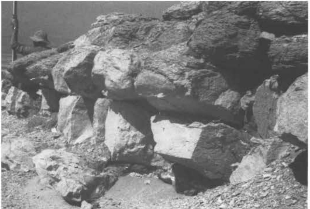
FIGURE 2b Inward inclining blocks. Pyramid of Seila. Photo I. E. S. Edwards.
