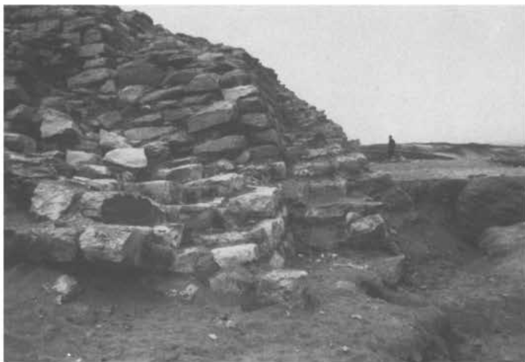
FIGURE 3 Flat and slightly inclining blocks. Pyramid of Seila. Photo C. W. Griggs.
