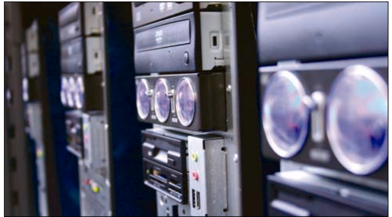
Tiny.com's manufacturing facilities have produced half a million PC system since launch
